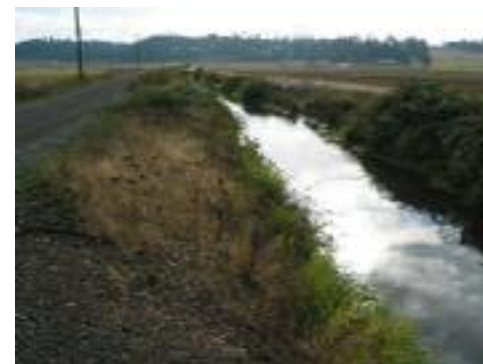
Figure 8. East/West Ditch (Ditch 6)
